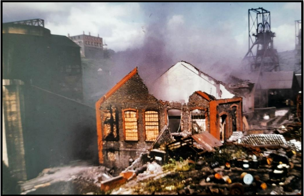
The demolition of Bargoed Colliery
